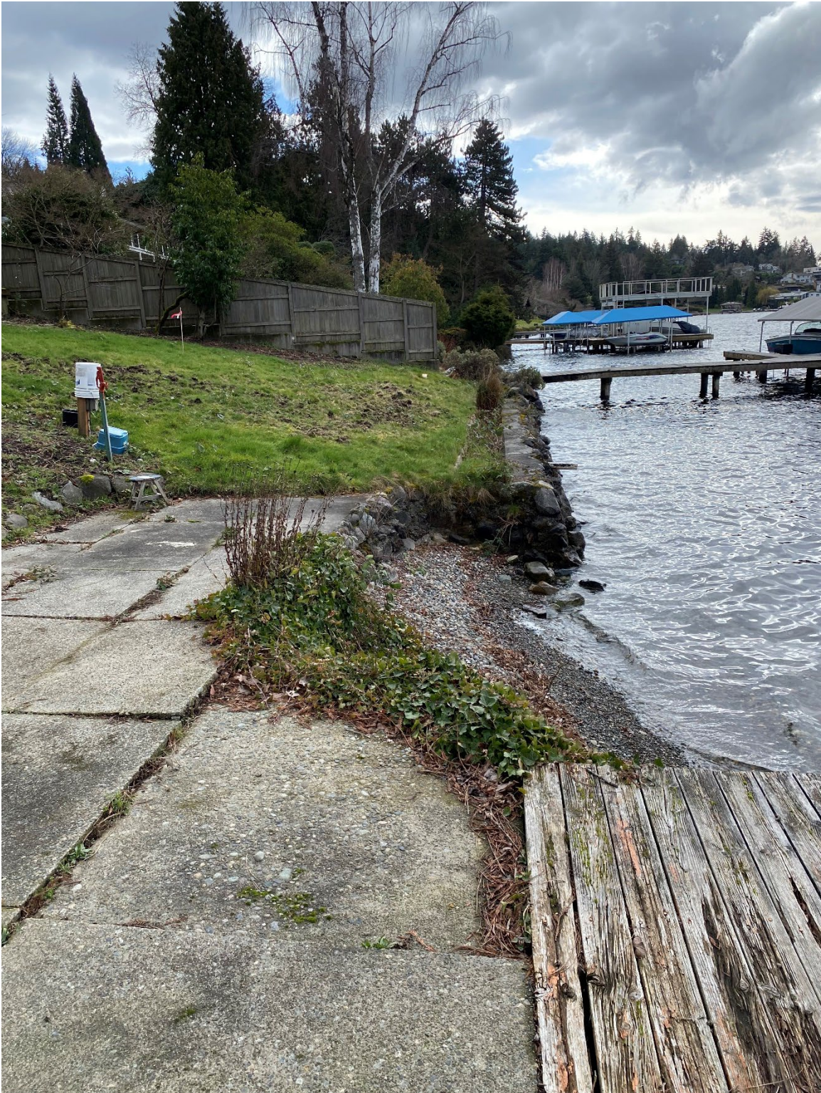
Typical view of shoreline looking south.
